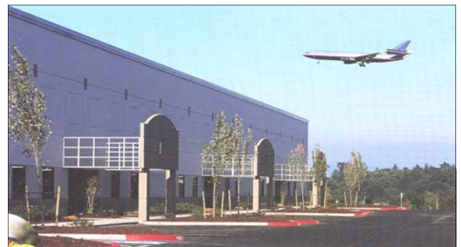
Premier Airfreight Facility in Seattle
