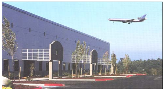
Premier Airfreight Facility in Seattle
